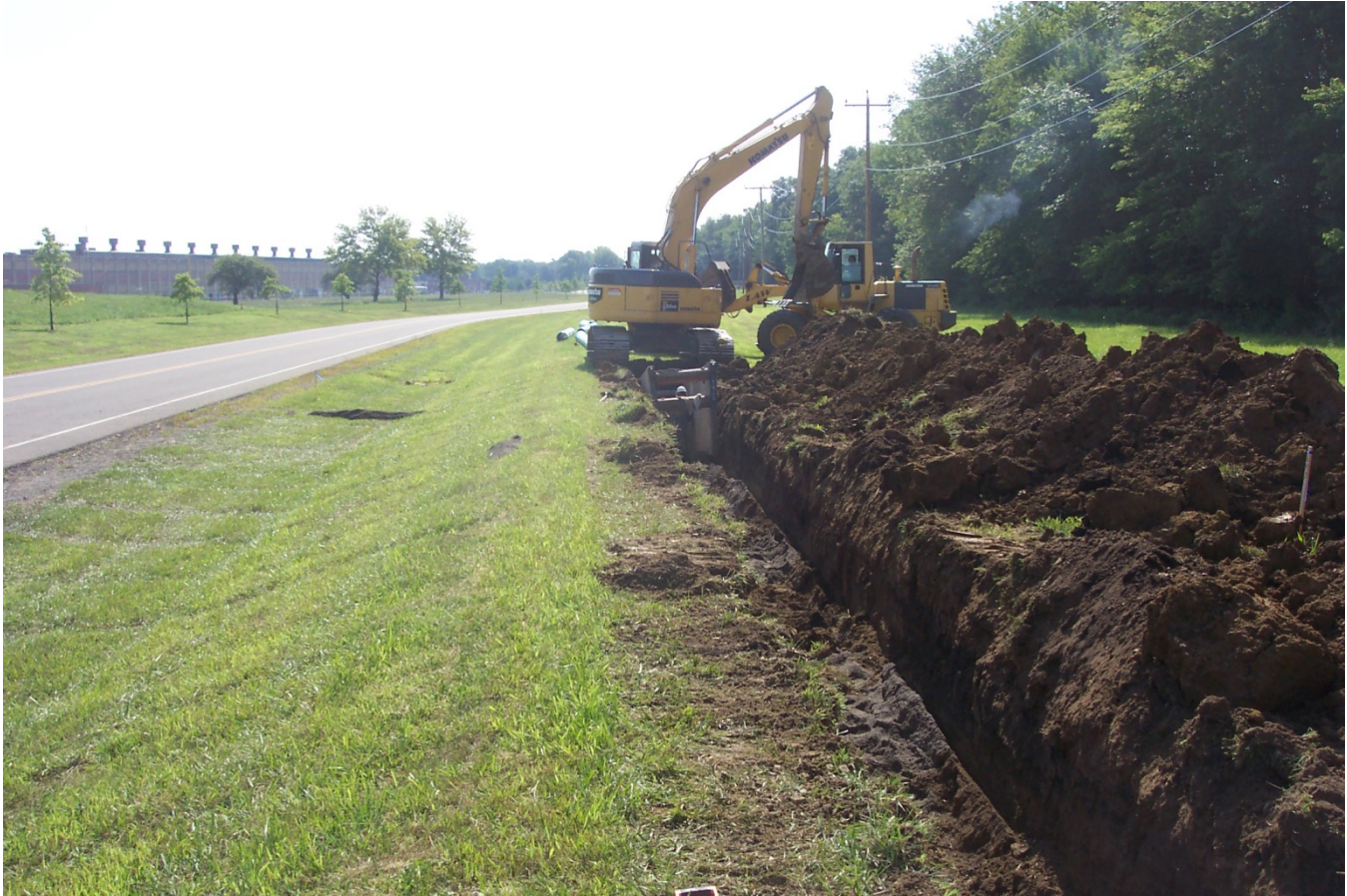
Figure 11. Overview of trench excavations.
