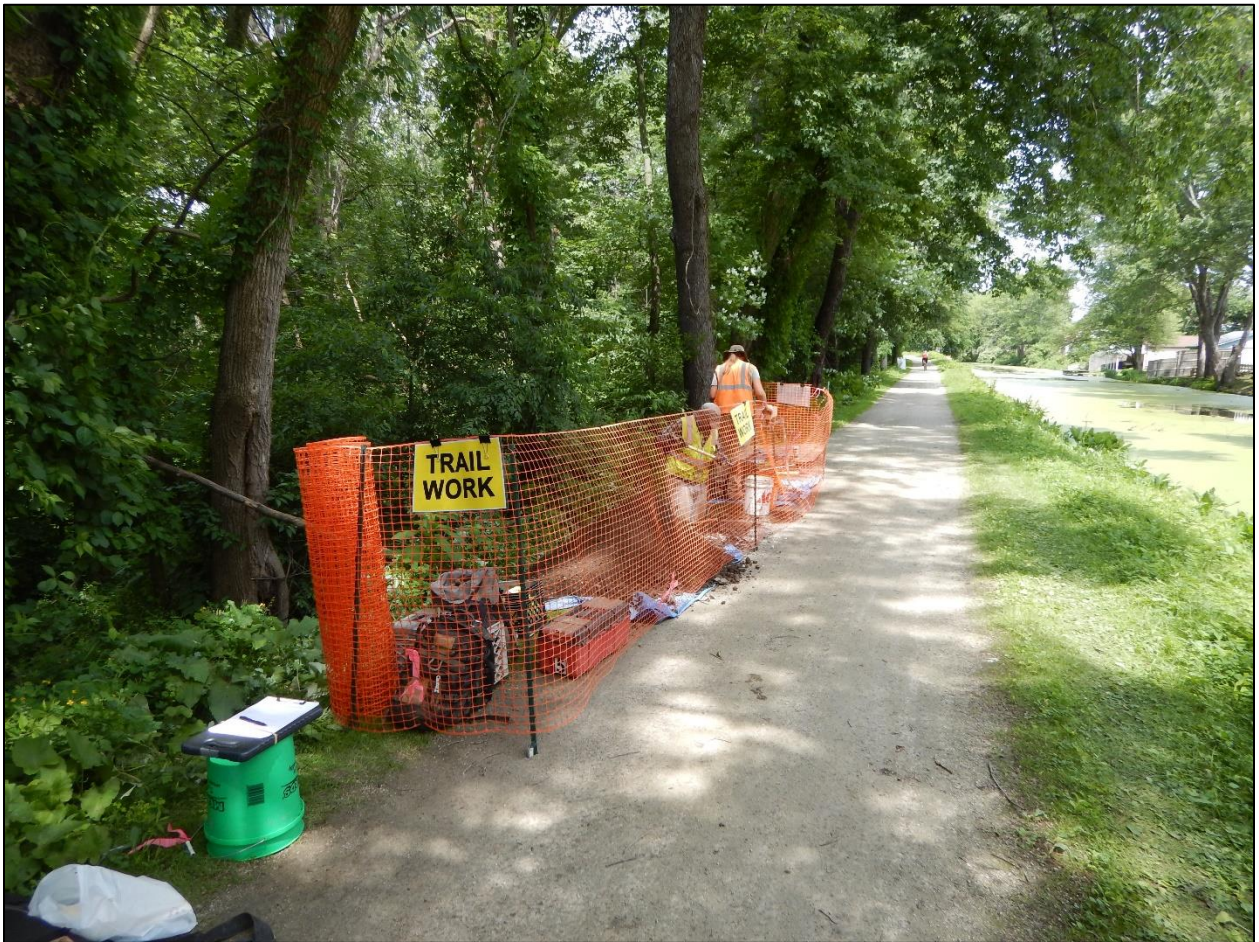
Figure 7. View facing west of unit excavation along the towpath.
