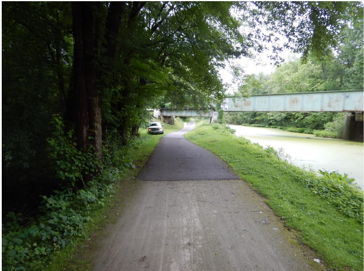
Figure 2. View facing west of a low spot along the Towpath Trail, where the trail height and towpath surface falls below the 100-year flood level.
